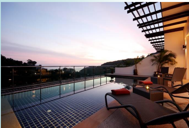
Completed Type A
