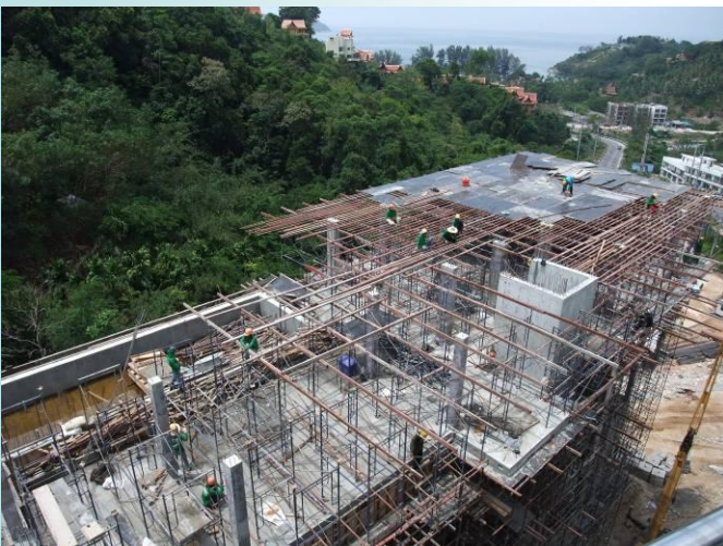
Building C1 penthouse roof preparations to complete superstructure
