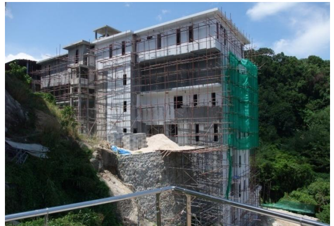
Building C1 – completing external painting
