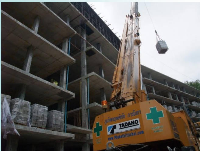
C Phase – Building C2 and C3 completed superstructure, bricklaying in progress
