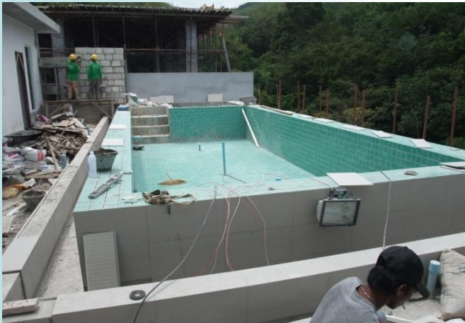
C1 Penthouse pool being tiled
