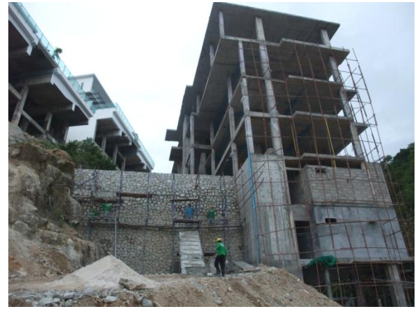
Building C1 – Retaining wall up to 2 nd floor completed
