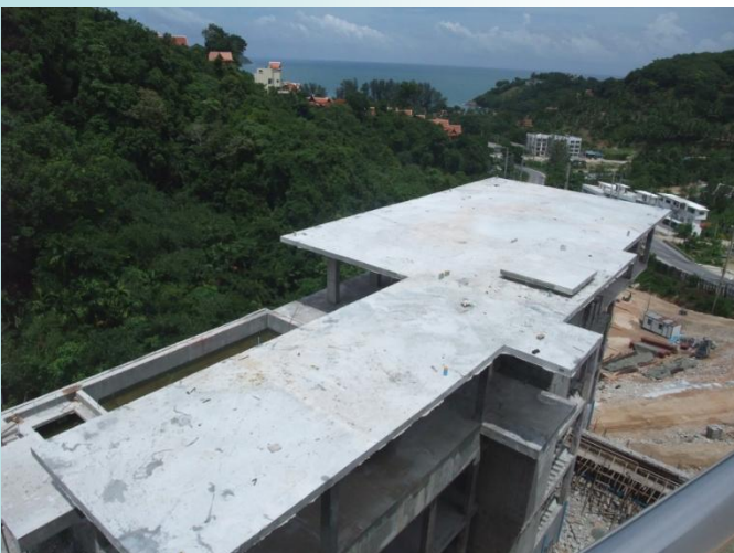
Building C1 superstructure completed – Penthouse rooftop
