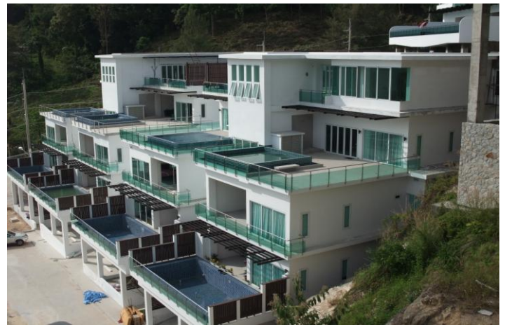
Building A3 and A4
