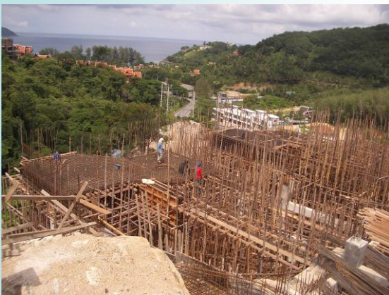
A5 swimming pool metal work foundation (early June 2008).
