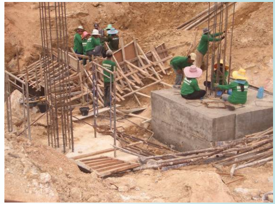
A1 – Piling and Footing construction (June 2008).
