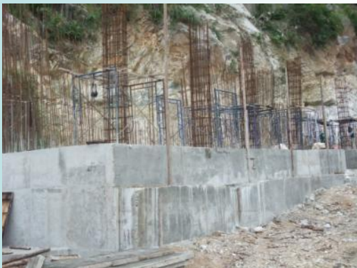
Phase C Ground works and formwork
