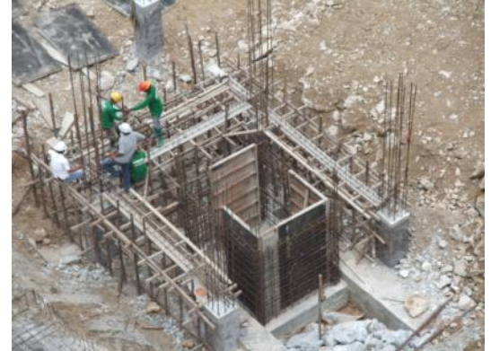
Building A4 elevator shaft
