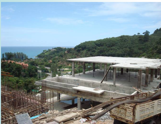
Building A5 completed Superstructure, on the left building A6 Superstructure underway.
