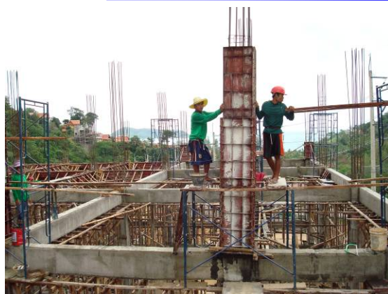
A1 - Completing Ground works.
