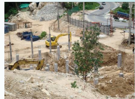
A4/A3 Footings and piling.
